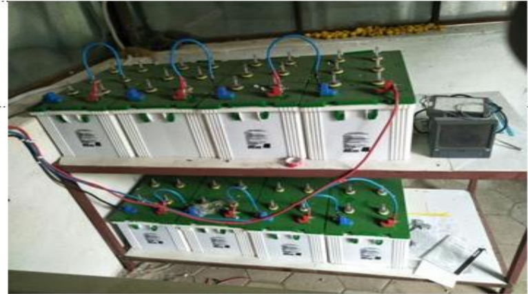
Solar Powered Street Light
